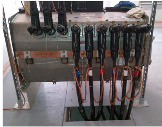
Figure 48 - Inside of SF6 underground switchgear
