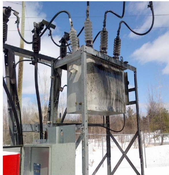
Figure 13 - Bridlewood Recloser Exploded Internally
