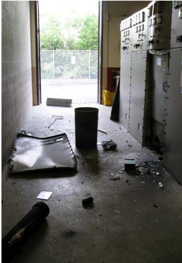
Figure 12 - Station Switchgear Explosion
