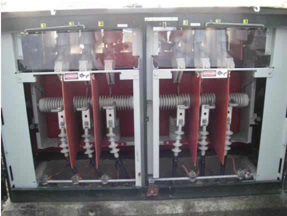
Figure 47 – Inside of air-insulated switchgear
